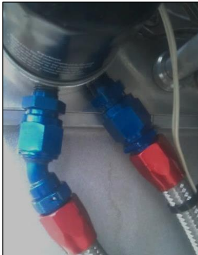
Photo No. 4: New hoses with screw-on fittings.
