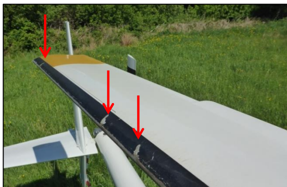
Photo No. 3: Damage on upper surface of main rotor blade leading edge
