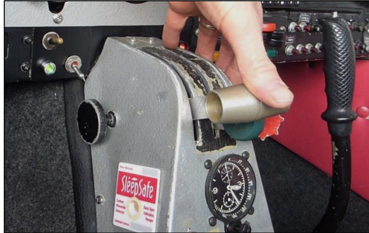
Photo No. 3: Throttle position required to actuate nose landing gear warning switch
